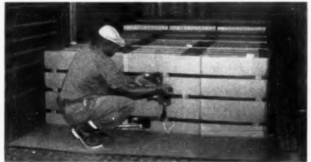
The straps on one of the end loads is here tightened.
